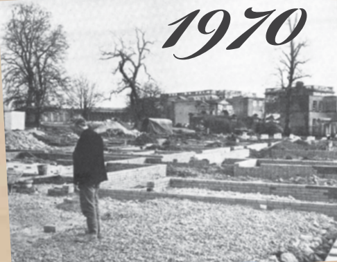
New Science Block under construction.
